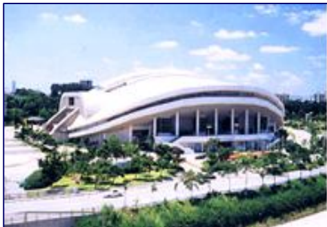
Olympic Swimming Pool
