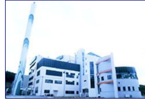
Paju MSW Sanitary Treatment Plant
