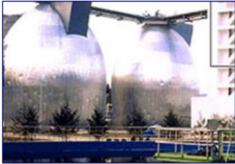
Masan Municipal Wastewater Treatment Plant
