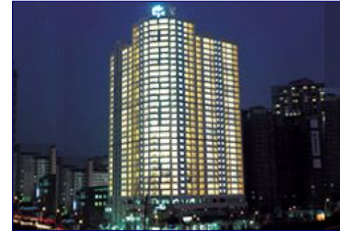
Kolon Hanulche in Bundang
