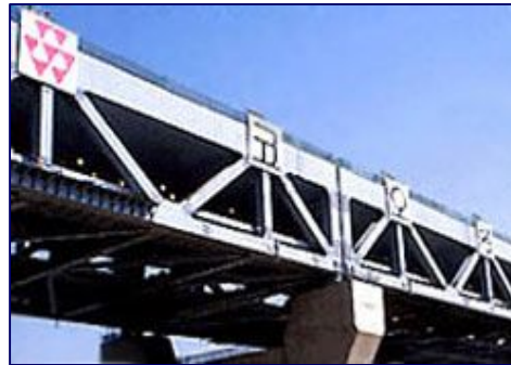
Incheon International Airport Expressway
